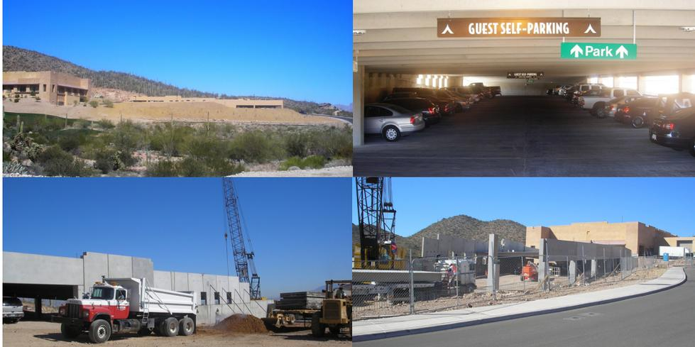
Design-build project consisting of 168 parking spaces in a multi-level garage adjacent to the Starr Pass Marriott for employee parking. The garage was built with precast concrete and included electrical, drainage, landscaping and irrigation.
